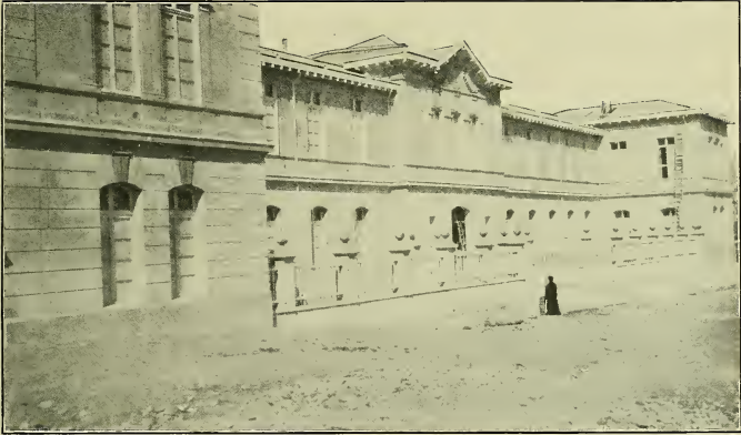
A. FAÇADE OF NEW NORMAL SCHOOL FOR GIRLS, LA SARENA, CHILE.
